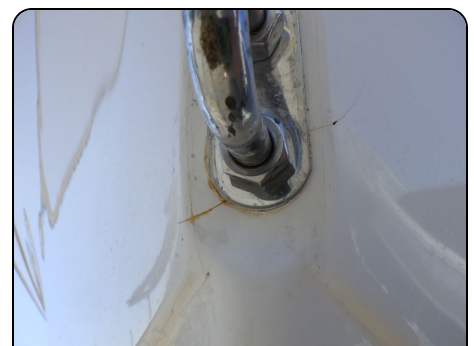
Bow tow eye with gel coat cracks
